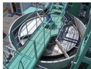
Super Dissolved Air Flotation Unit
